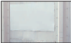
Self-adhering Natural Aluminum Panel Patch Repair
